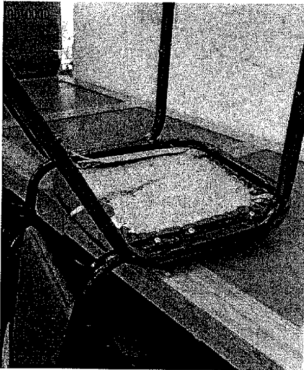
13 chairs with broken seat boards
